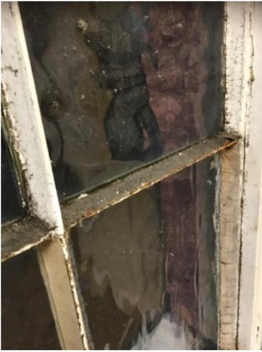
The windows on the Bowling Green side have now all been fitted with temporary shutters and deglazed. It takes many more hours of work per window to strip them down to the metal and to repaint them in preparation for reglazing. However, once at this point they work perfectly and with good ongoing maintenance have
