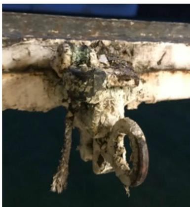
(long gone) spring loaded brass catches of the opening 'hoppers' were completely seized with paint and the hoppers stuck shut or slightly open and gummed up with silicon. With the help of paint stripper and a wire brush on a drill it takes about 3 hours
